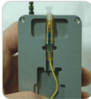
5. Inserting cable(fiber) until bending occurs(important)
