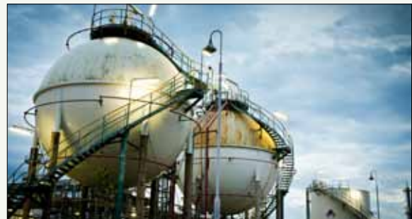
Korea Gas Corporation Substation 21 in Pyeongtaek
